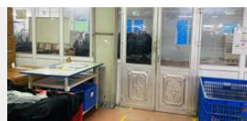
Sliding door of dehumidifier room workshop 2 was replaced by side hung door
