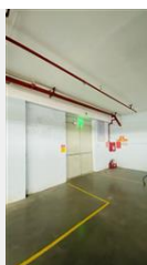
Enclosure for stair at workshop 5-6 , 2nd floor
