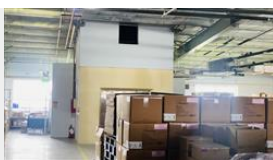
Enclosure for stair at workshop 5-6 , 3rd floor
