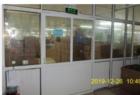
Sliding door on exit path dry room workshop 2
