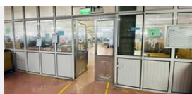
Sliding door at dehumidifier room workshop 2 was replaced by side hinged door
